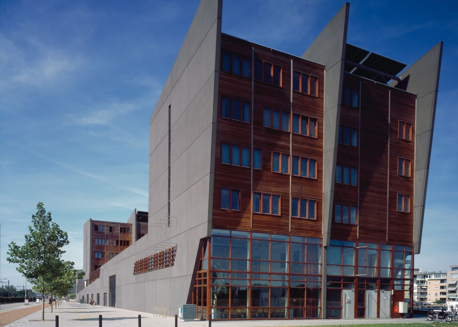
The vast town hall, with its four distinctive towers built from integrally colored concrete, rises up from the wharf.
